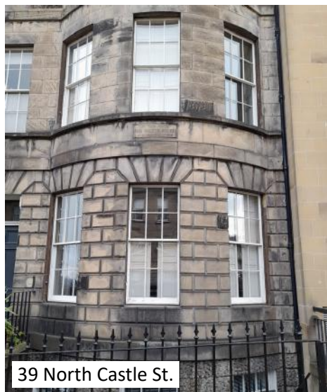
Sandstone replacement, Contini (detail)
