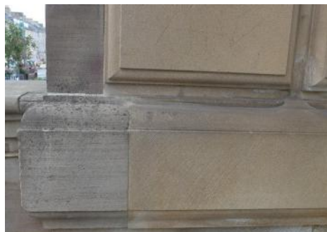
Sandstone replacement, Contini (detail)
